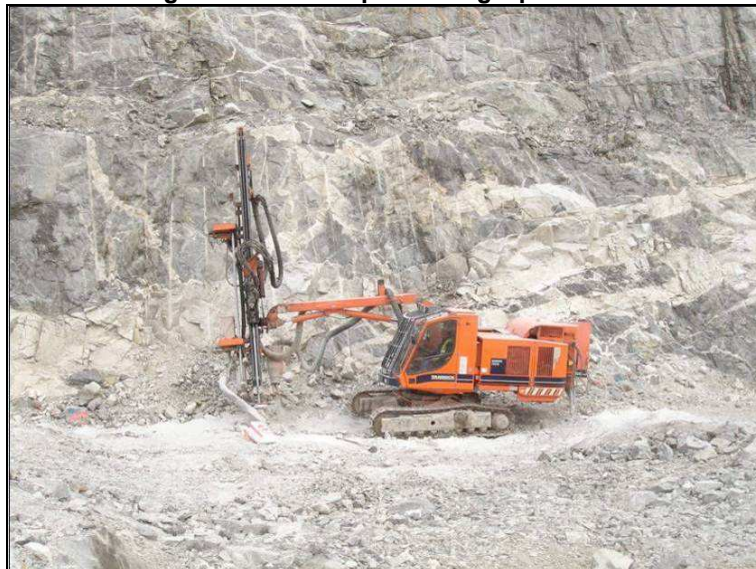
Figure 16-2. Pre-Split Drilling Operations
