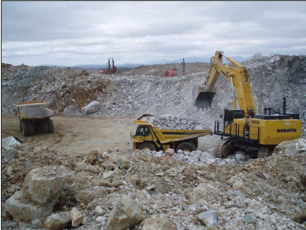
Figure 16-4. Mucking Operations at Los Santos Sur
