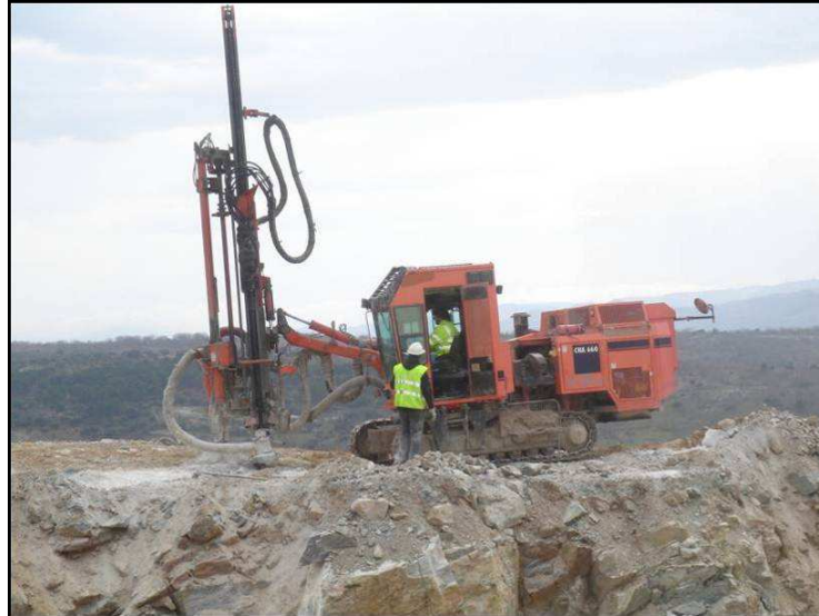
Figure 16-1. Blasthole Drilling Operations
