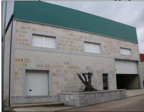
Figure 11-6. Daytal's Core Shed and Logging Facility
