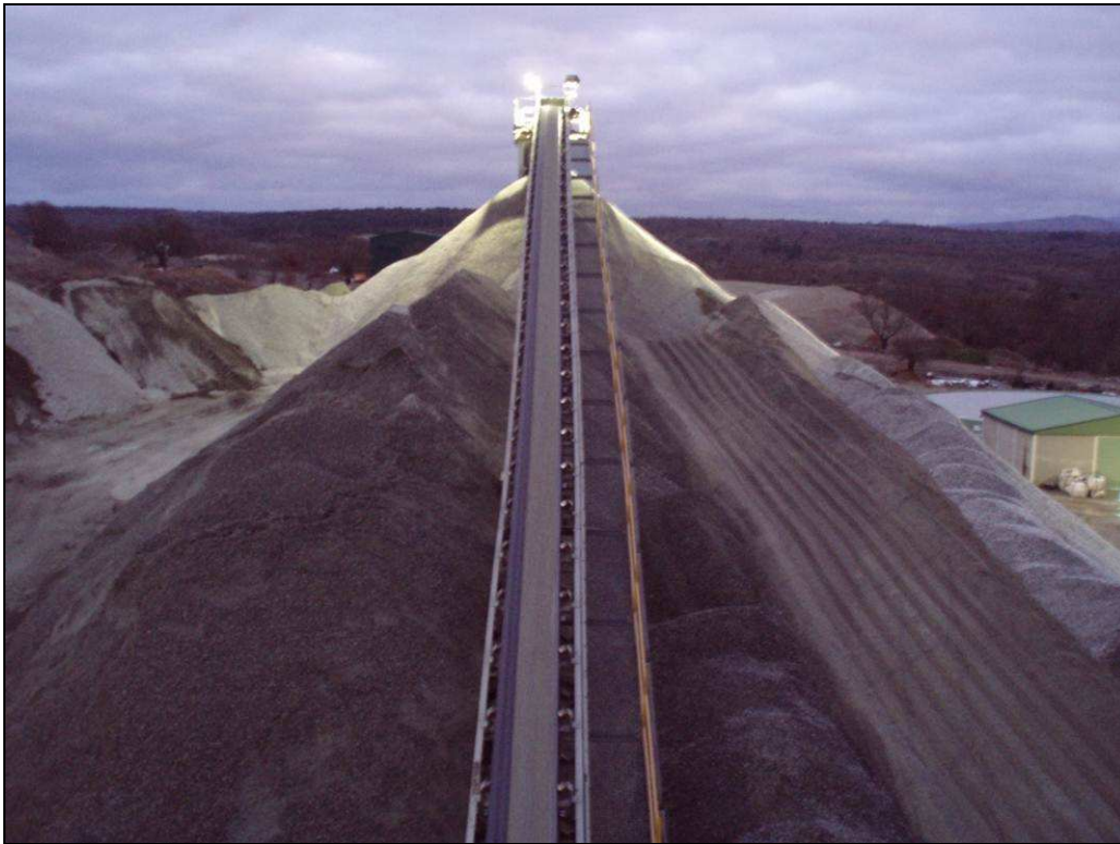
Figure 13-1. Intermediate Crushed Stockpile.
