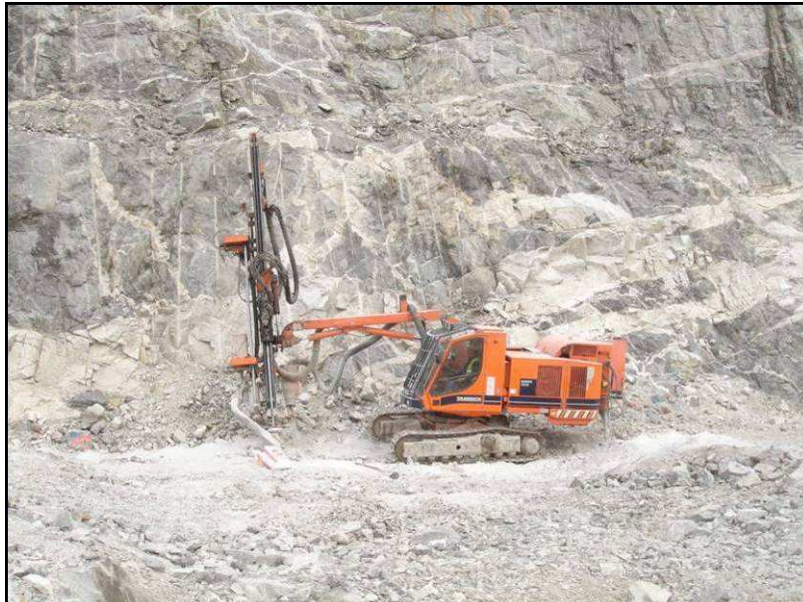
Figure 16-2. Pre-Split Drilling Operations
