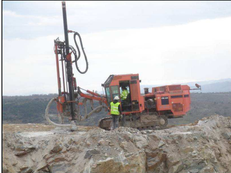
Figure 16-1. Blasthole Drilling Operations
