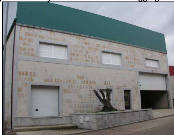
Figure 11-6. Daytal's Core Shed and Logging Facility
