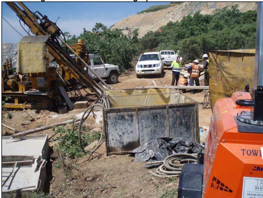
Figure 9-1. Diamond Drilling Operations at Los Santos
