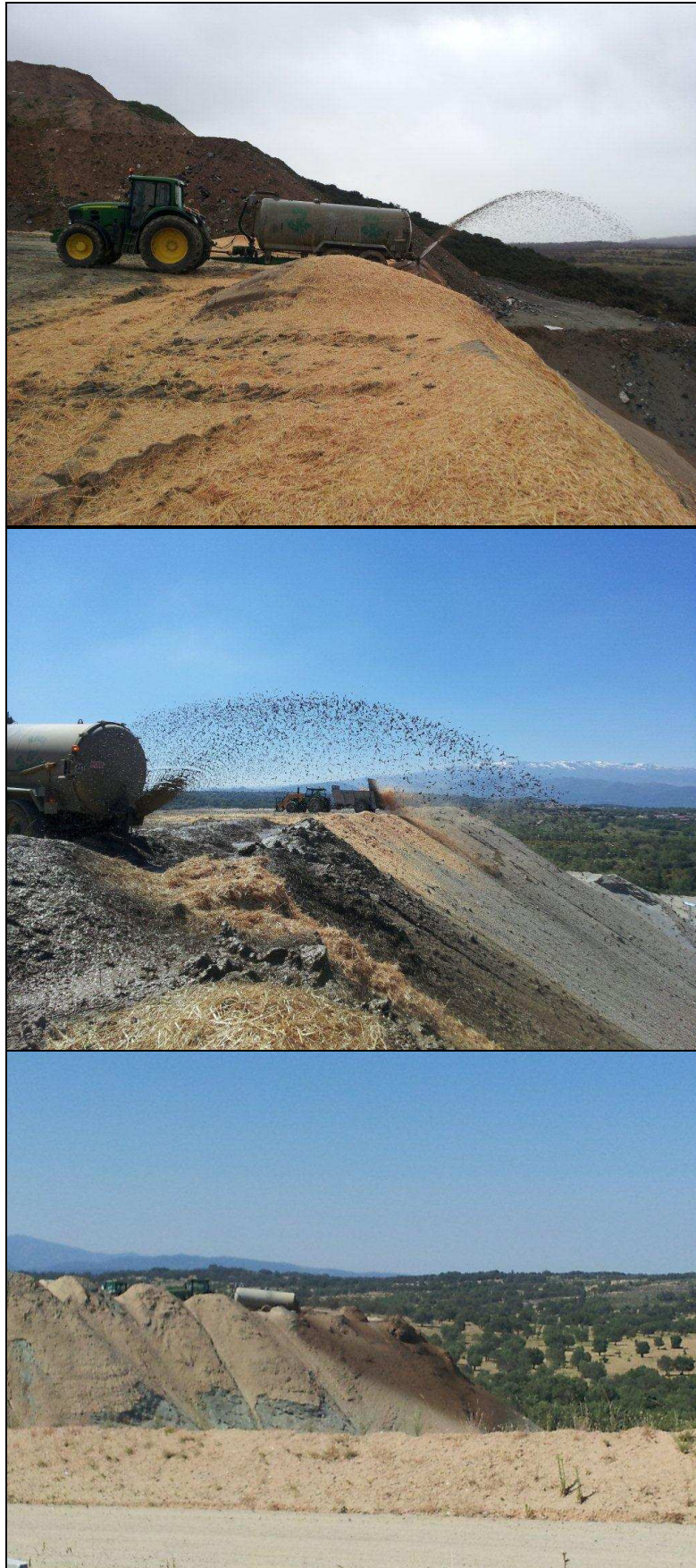
Figure 17-3. Dust Control System
